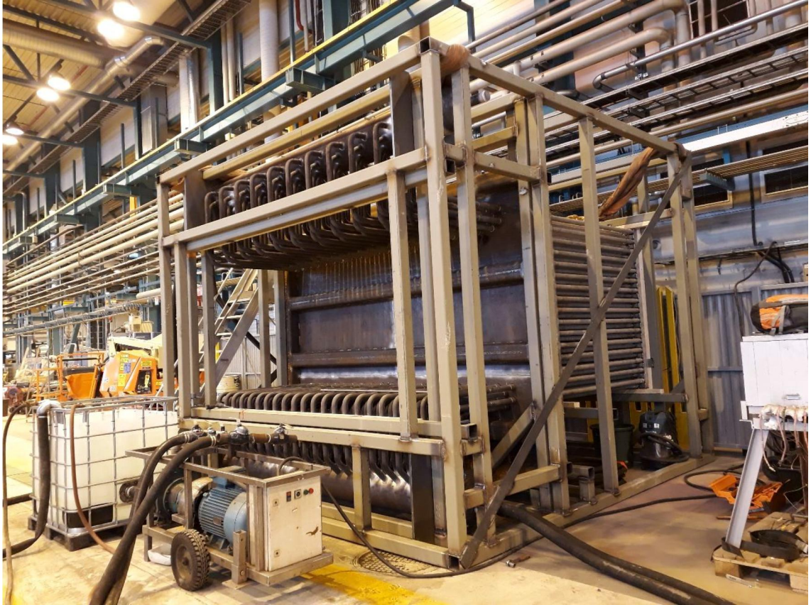
Figure 12. Chemical cleaning of Valmet's superheater executed by Enerkem Oy.
