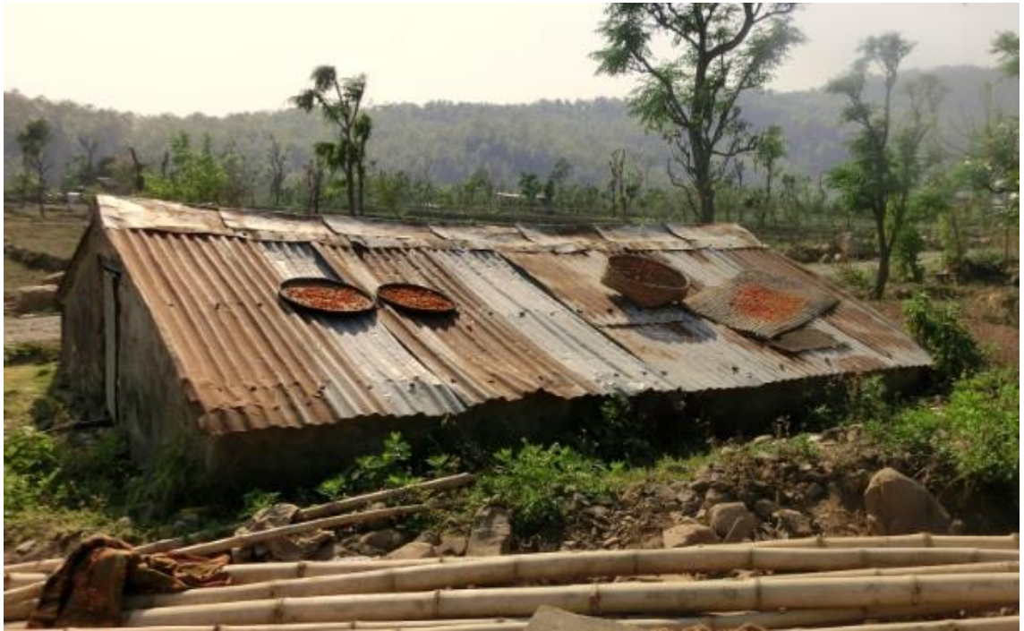
Figure 15. The already old reservoir tank of the Ranibel scheme.
