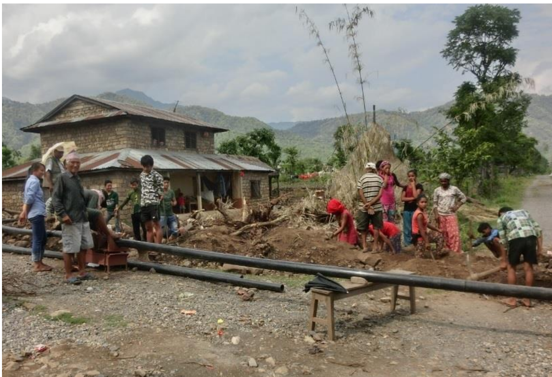
Figure 13. Villagers reconstructing a distribution line in Aaptari.
