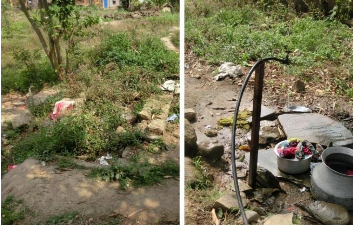
Figure 16. From Mirtung khola scheme, on the left: a broken or abandoned tap stand. On the right: a public tap without a proper tap stand.
