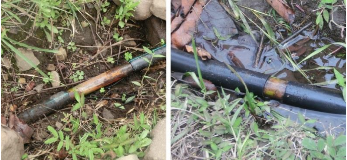
Figure 23. Some pipelines that have been fixed with bamboo.
