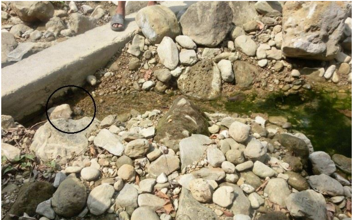
Figure 25. The intake of the Mirtung khola scheme with the intake pipe circled in the picture. A lot of algae was growing in the river close to the intake.
