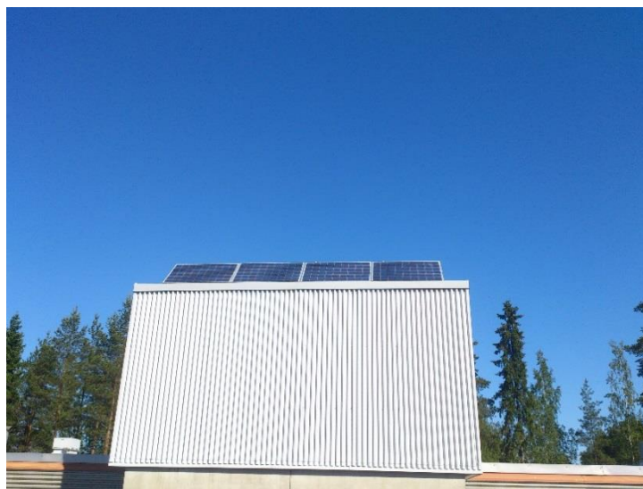
Figure 5.14 PV module string at the highest point of the TUT PV power plant.
