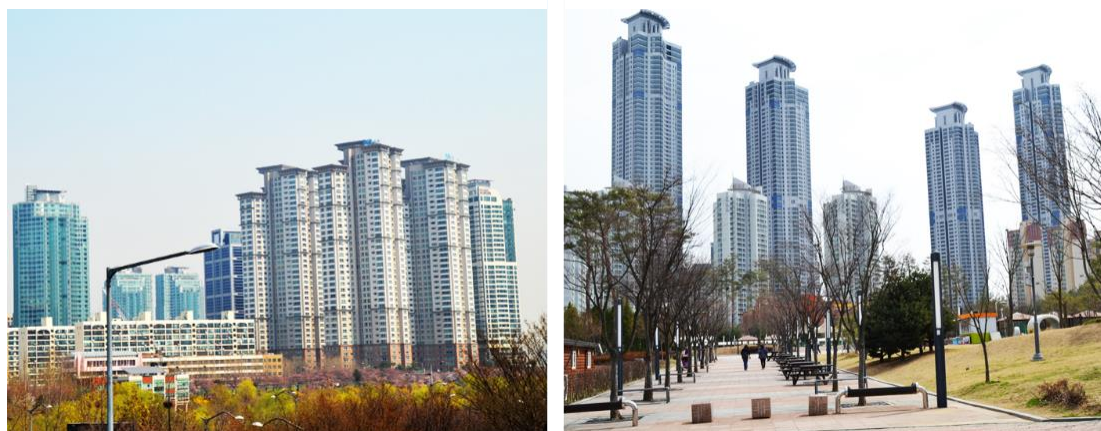
Figure 6. Block of Flats in South Korea
