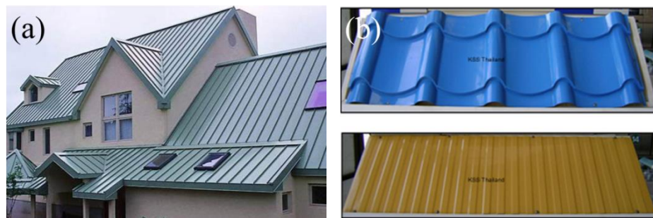
Figure 4. Sheet steel application in buildings. A house with sheet steel roofing (a) two types of corrugation sheet steel (b) [29]
