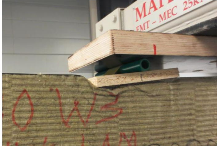
Figure 35: Wrinkling failure next to the load plate
