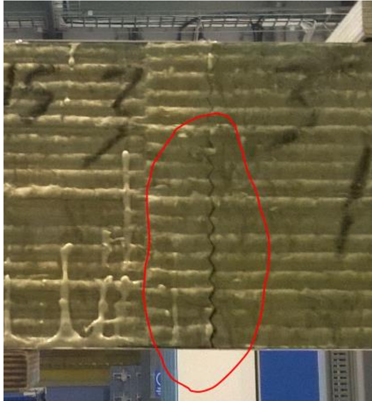
Figure 46: The gap in the mechanical connection
