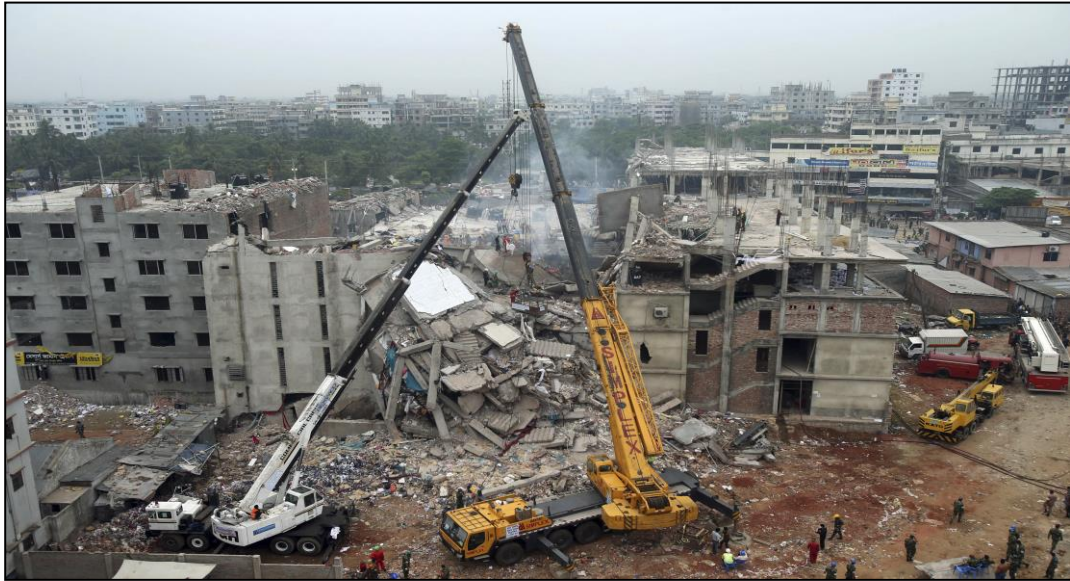
Figure 3:2 Debris of collapsed garment factory Rana plaza garment factory (Halkias, 2015)
