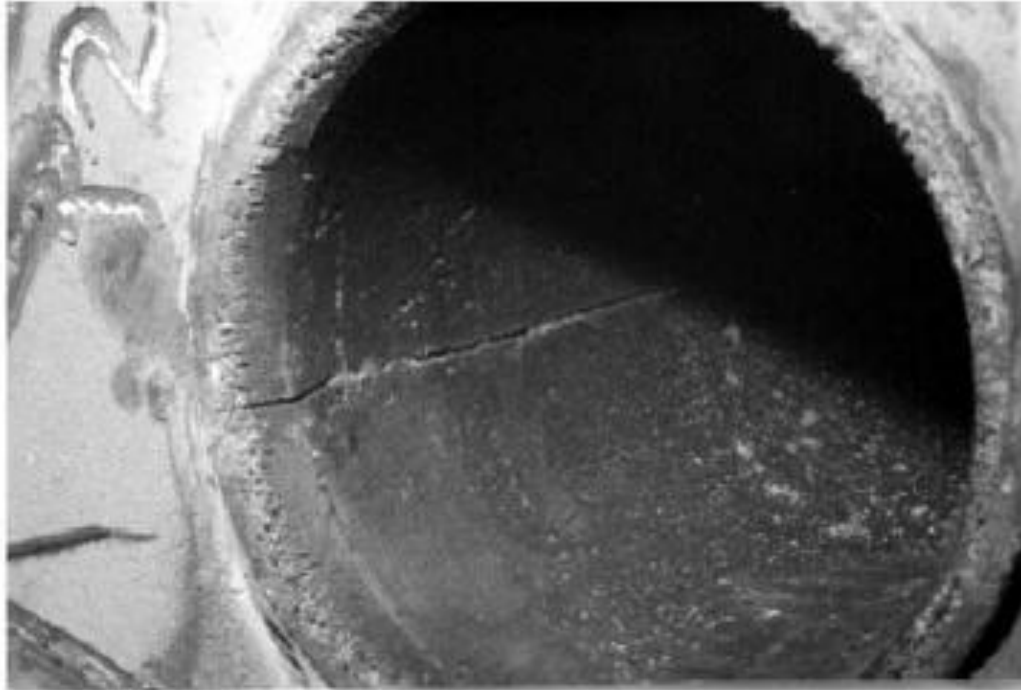
Figure 3-4 Longitudinal cracking of steam drum downcomer nozzle. Source: (Coleman, 2004)
