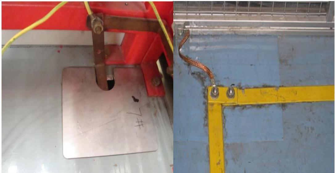
*Figure 11. Earthings in testing areas. [15]*
