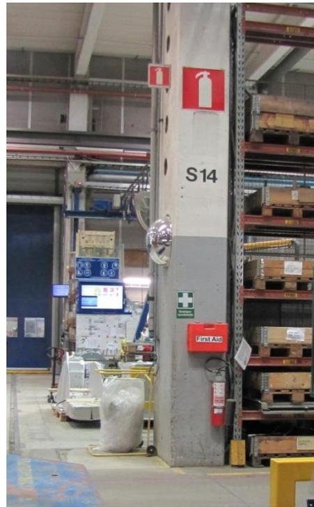
*Figure 15. A sign telling place for firefighting equipment*
