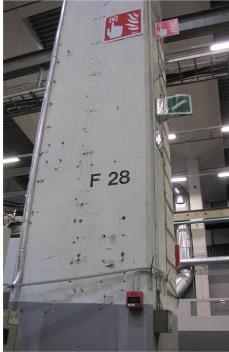
*Figure 14. Signs telling a place for a call point in case of a fire.*
