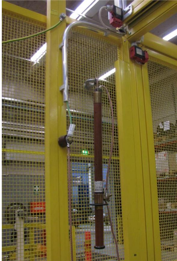
*Figure 12. Portable earthing device*
