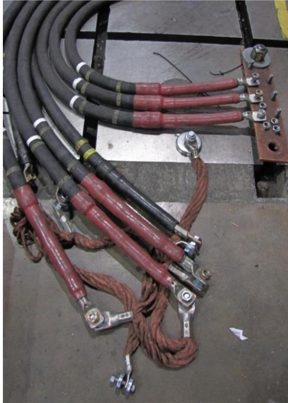
**Figure 18.** *Unused cables earthed in test area.*
