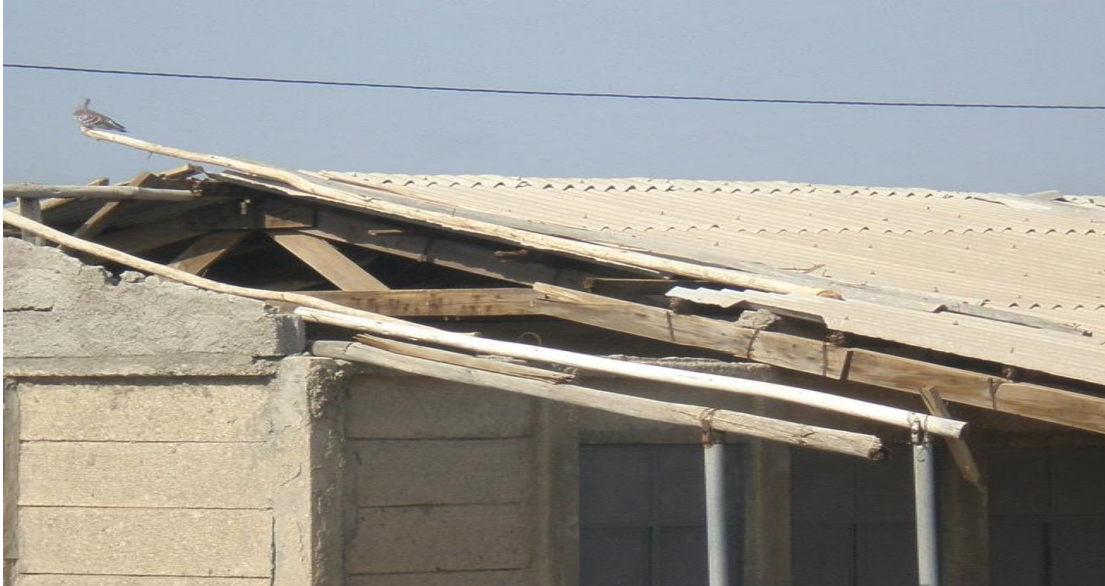
Photo 4: Serdo primary school in Afar with part of the room taken by the desert wind (built by SIDA in 1971) Source: Photo by the researcher during field survey
