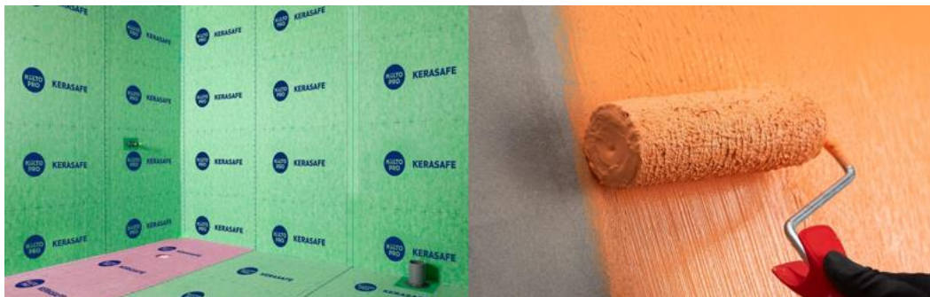
Figure 9. Use of waterproofing films and waterproofing membrane [139].
