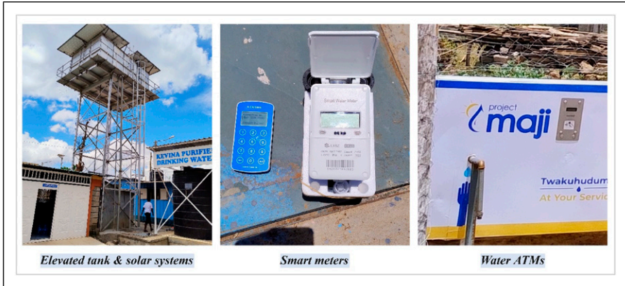
Figure 7. Water systems, smart meters, and water ATMs used by small-scale water operators.
