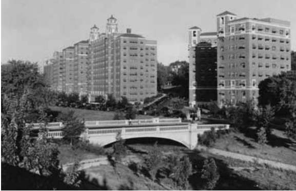
Figure 6: A photograph of the apartment buildings along Brush Creek. With their lush surroundings and automobile accessibility, these buildings were integrated into the Plaza's new spatial program. Courtesy of MVSC-KCPL.
