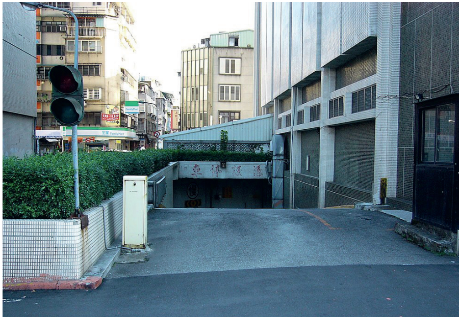
fig. 3. Passage to an underground parking lot.
