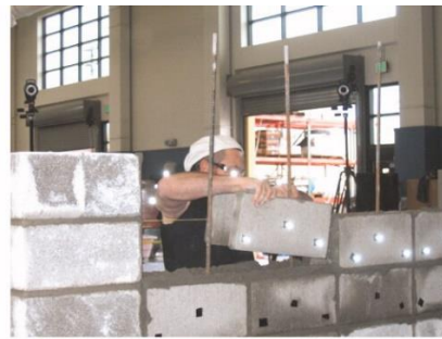
(b) Placing H-block
