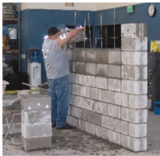
(a) Placing conventional CMU
