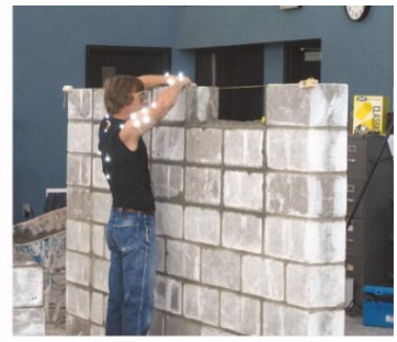
(c) High-lift grouting
