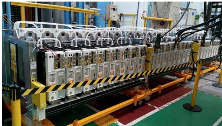
**Figure 5.** MMC STATCOM valve module [11]
