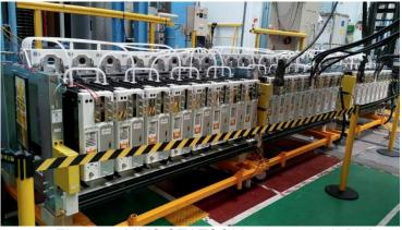
Figure 5. MMC STATCOM valve module [11]
