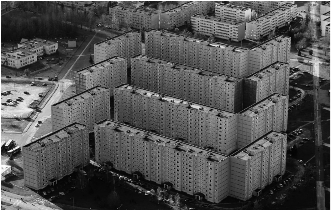
Figure 8. oPEN Lab pilot area in Tartu – three 9-storey apartment building will be renovated by using prefabricated insulation elements (photo Andres Tarto, 2013. EAM Fk 19856).
