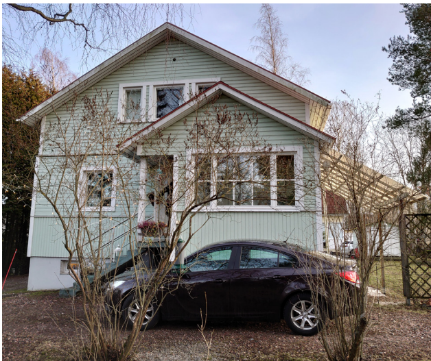
Figure 13 The frontman's house on the plot, picture taken from the road
