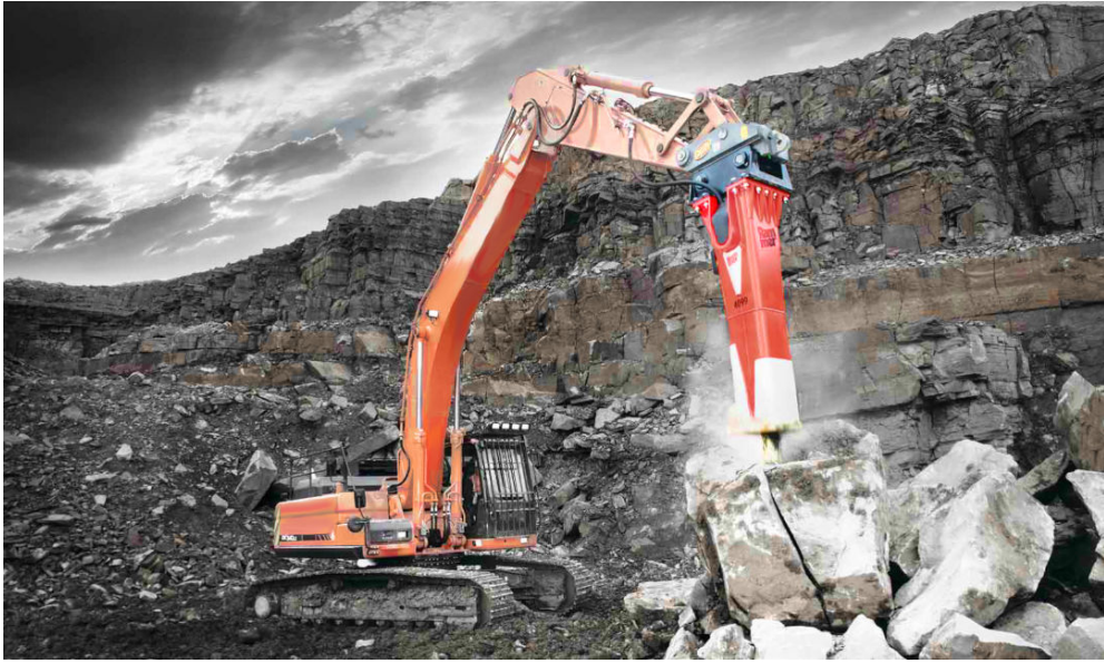
Figure 4.1 Hydraulic impact hammer mounted on an excavator in an open-pit mine.
