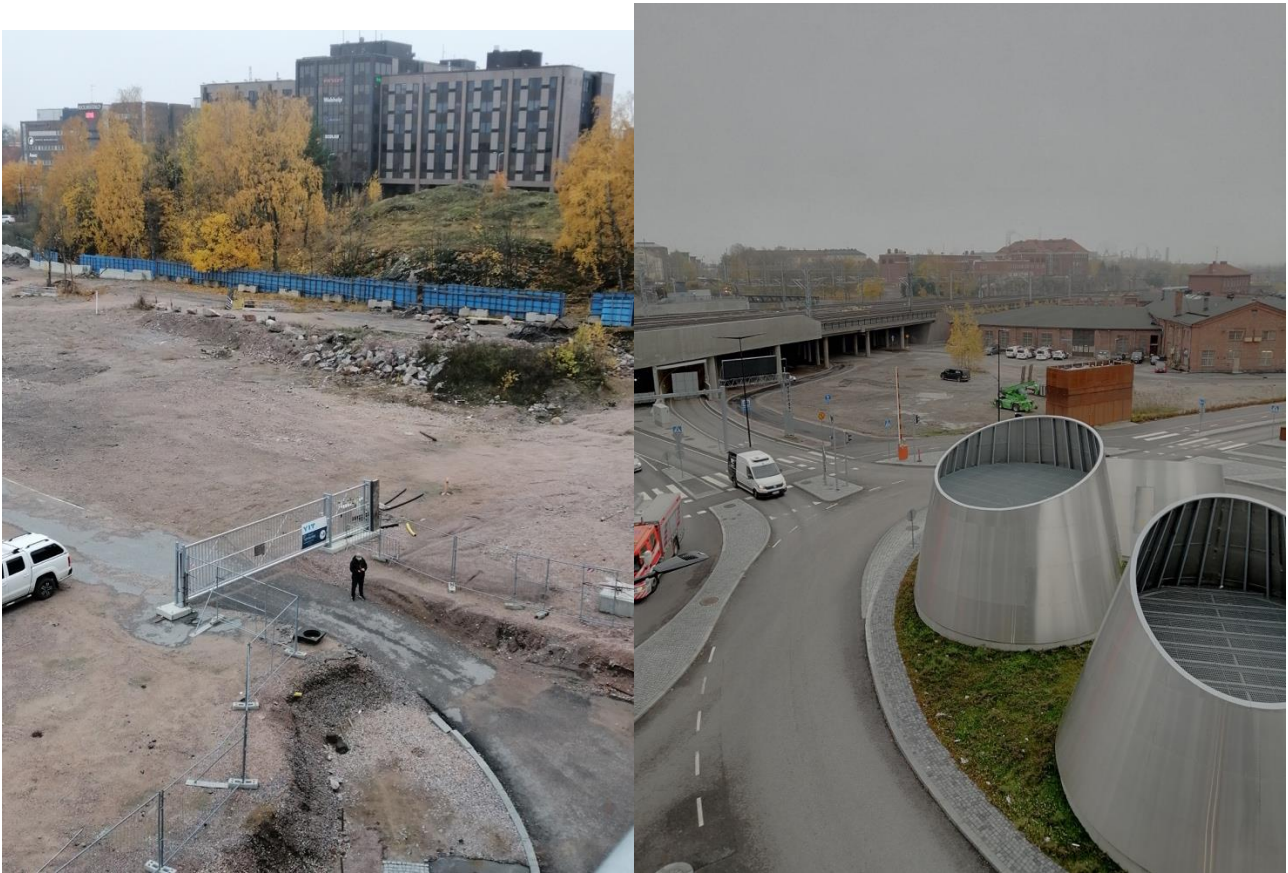
Figure 4: The intersection in Pasila
