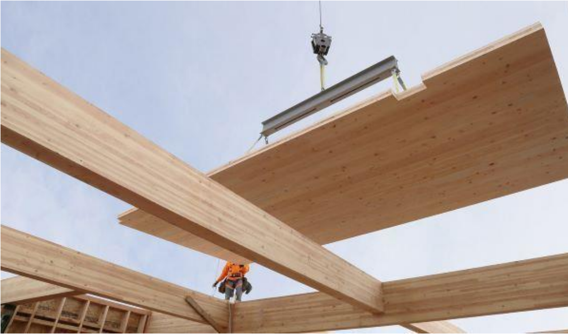
Figure 10. CLT ceiling panel assembling (©Wigo.info).
