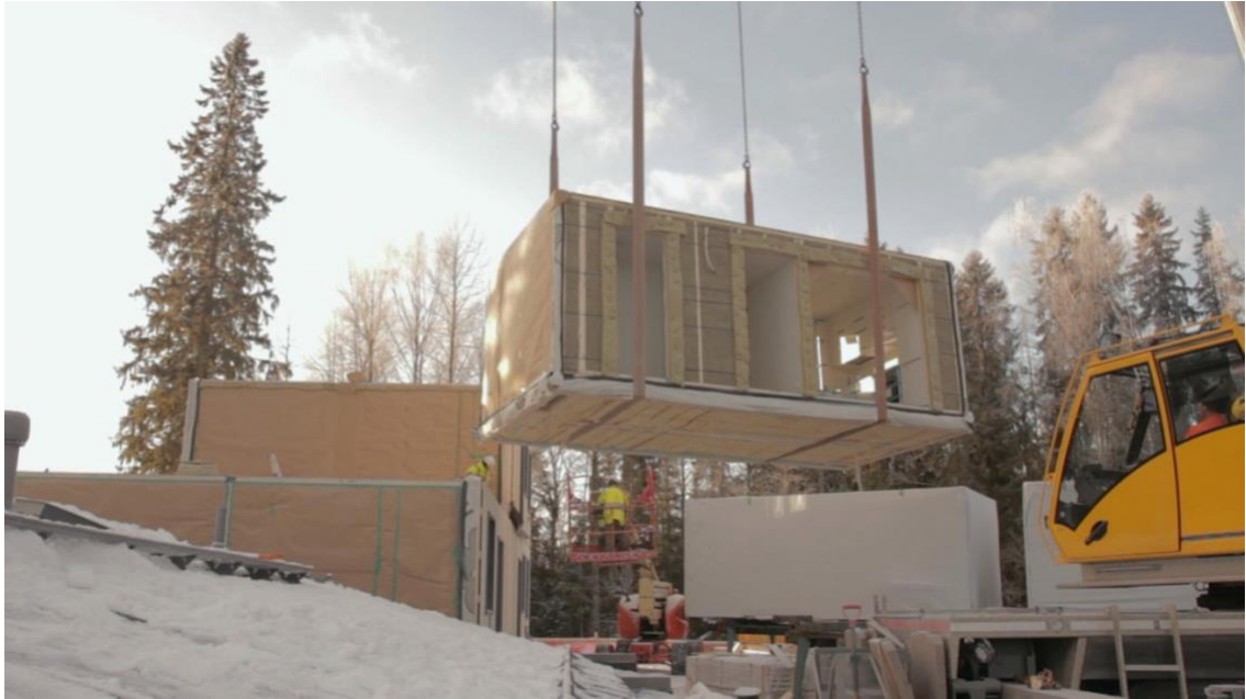
Figure 11. Modular element from massive timber elements (©Skanska).
