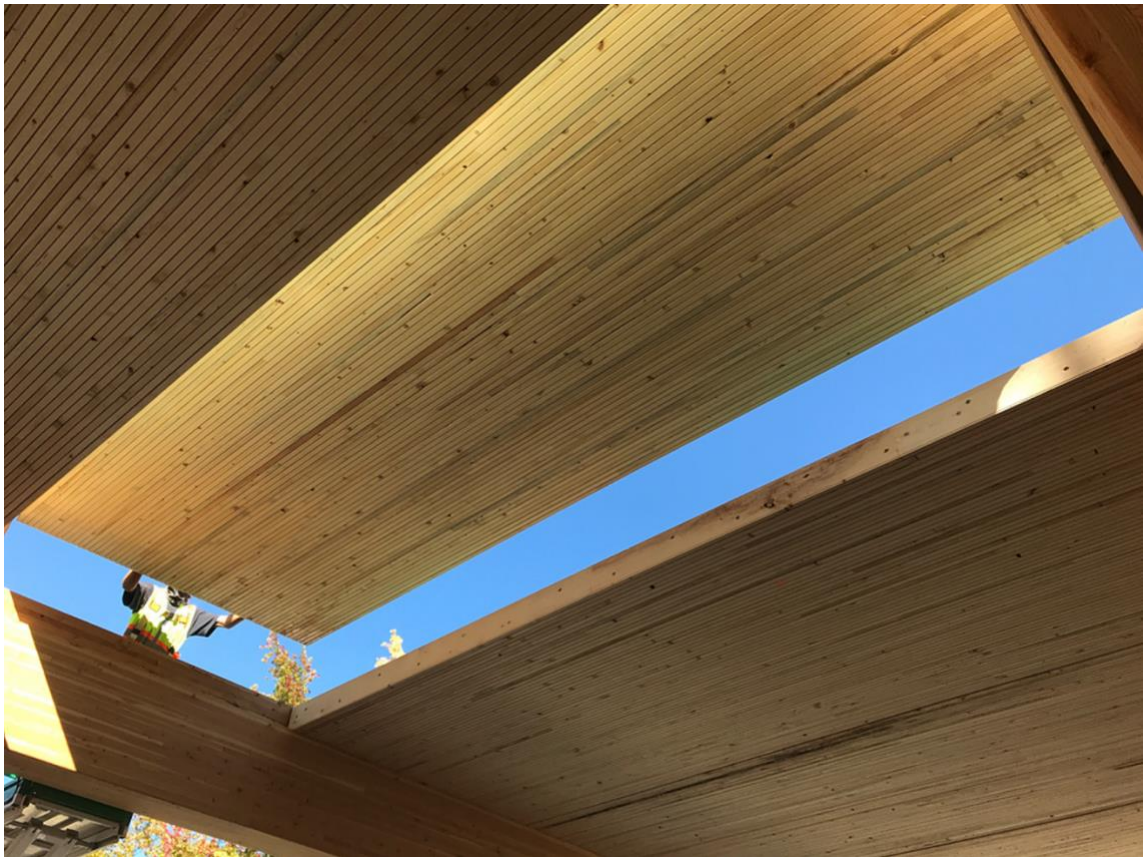
Figure 7. Dowel laminated timber ceiling panel in Lakeview office building (©StructureCraft).
