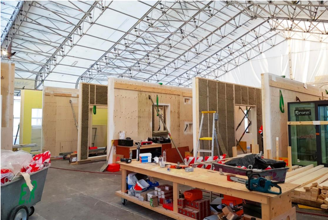
Figure 30. Equipping of the elements in-site (©Arcadia).
