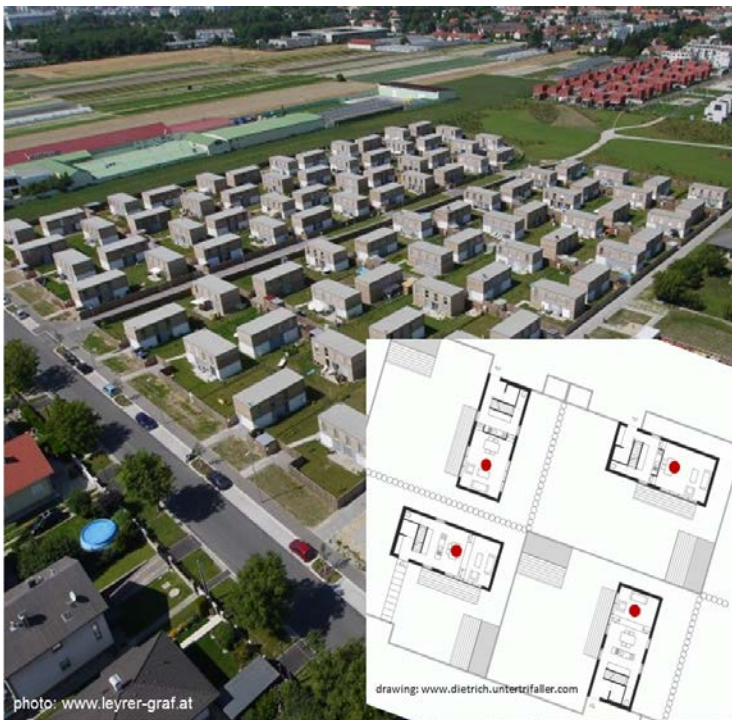
Figure 1. Residential area with similar single family houses. The location of the temperature and humidity sensors are shown in the drawings.
