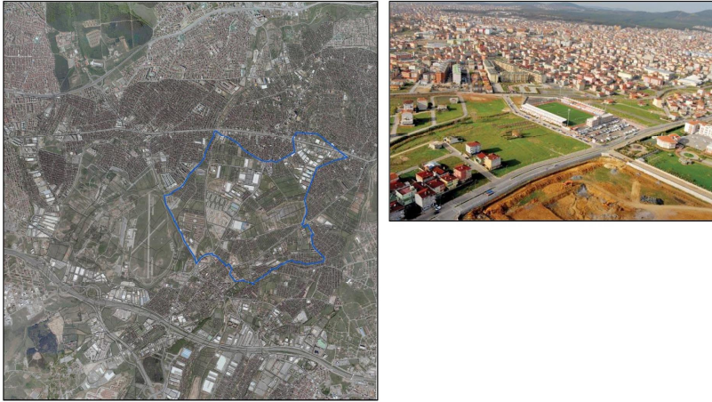
Figure 5: Case study area in its close vicinity (2014) and a recent picture of case study area showing urbanized small size land plots in background with some vacant lands in transition (foreground).
