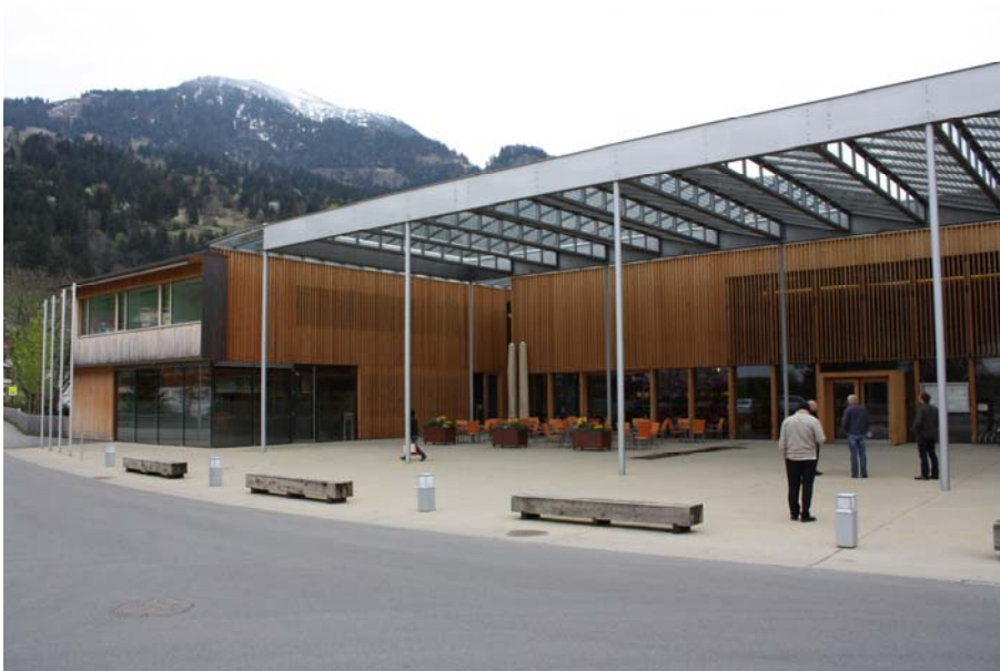
Figure 13. An office building in Austria with solar cell panels integrated in the roofing above the square area. Solar energy is not widely used in Norway, perhaps it will be in the future years to come?
