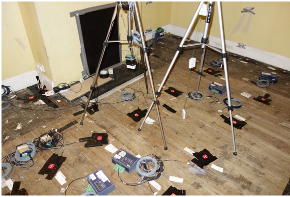
Fig. 3. Post-bead insulation with monitoring instruments in place.
