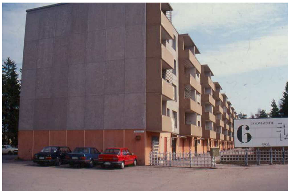
Figure 2 – Case building in 1994 during first condition investigation.
