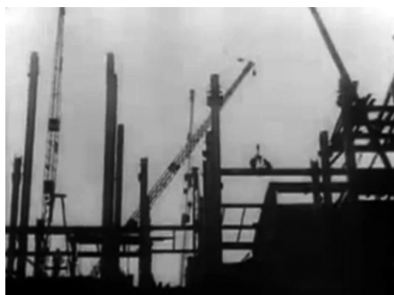
Fig. 1: Manhatta ; iron beams viewed from below.
