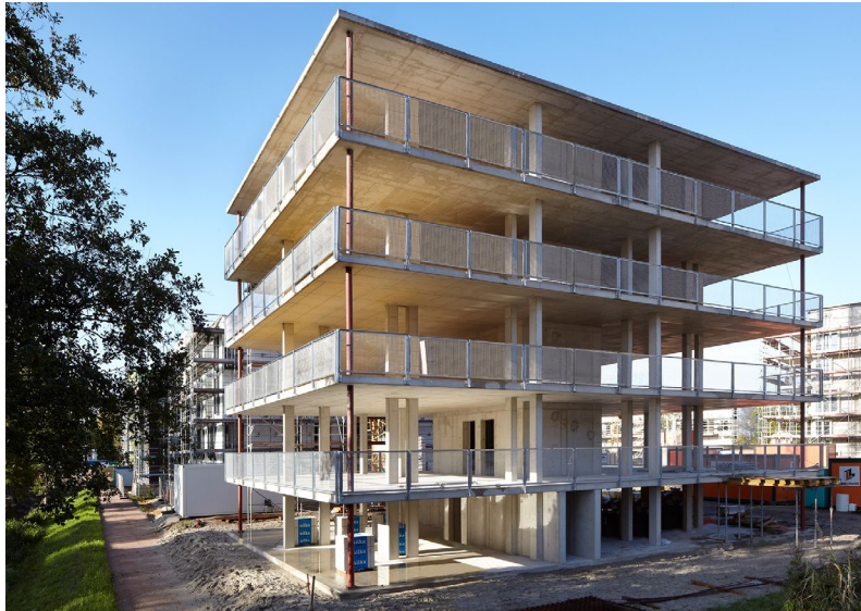
Completion of the base structure, 2013
