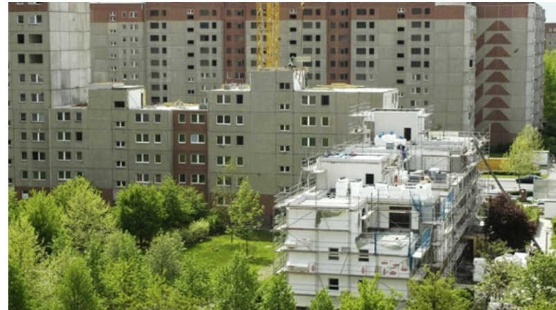
Berlin Ahrensfeld during the renovation in 2008
