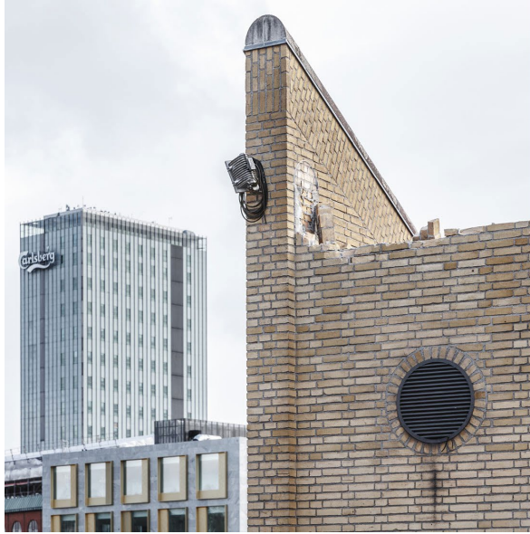
The disassembly of the an brick wall
