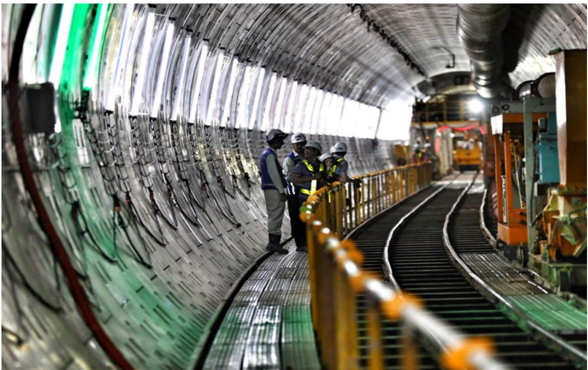
Picture 4: Benthanh Metro station is currently under construction
