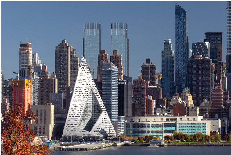
Figure 3.29: The VIA 57 west (2016), BIG. Manhattan, New York City, NY, USA. The building can appear as an exaggerated version and a caricature of fengshui's principles. As every feature is formed rather excessively, it turns against the residents. The form cast's massive shadow in the back, as well as the courtyard. Nearby water is far too vast and therefore windy. Topography is replaced by massive skyscrapers, etc.
