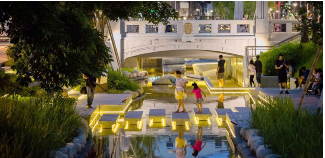
Figure 2.12: Xinsheng Green Waterway (新盛綠川水岸廊道), Taichung, Taiwan. A 610 meter restored section of the Green River, was built for improving air quality in 2018 and is now a popular place for leisure among the residents.
