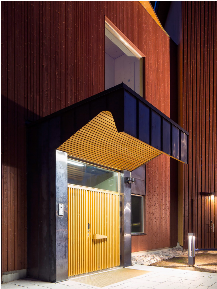
Figure 2.5: Finnish Nature Center Haltia (2013) by Lahdelma & Mahlamäki. Espoo, Finland. Combinations of wood and metal, light and dark tones, warm and cold colors, are all successfully present, and in dual harmony.
