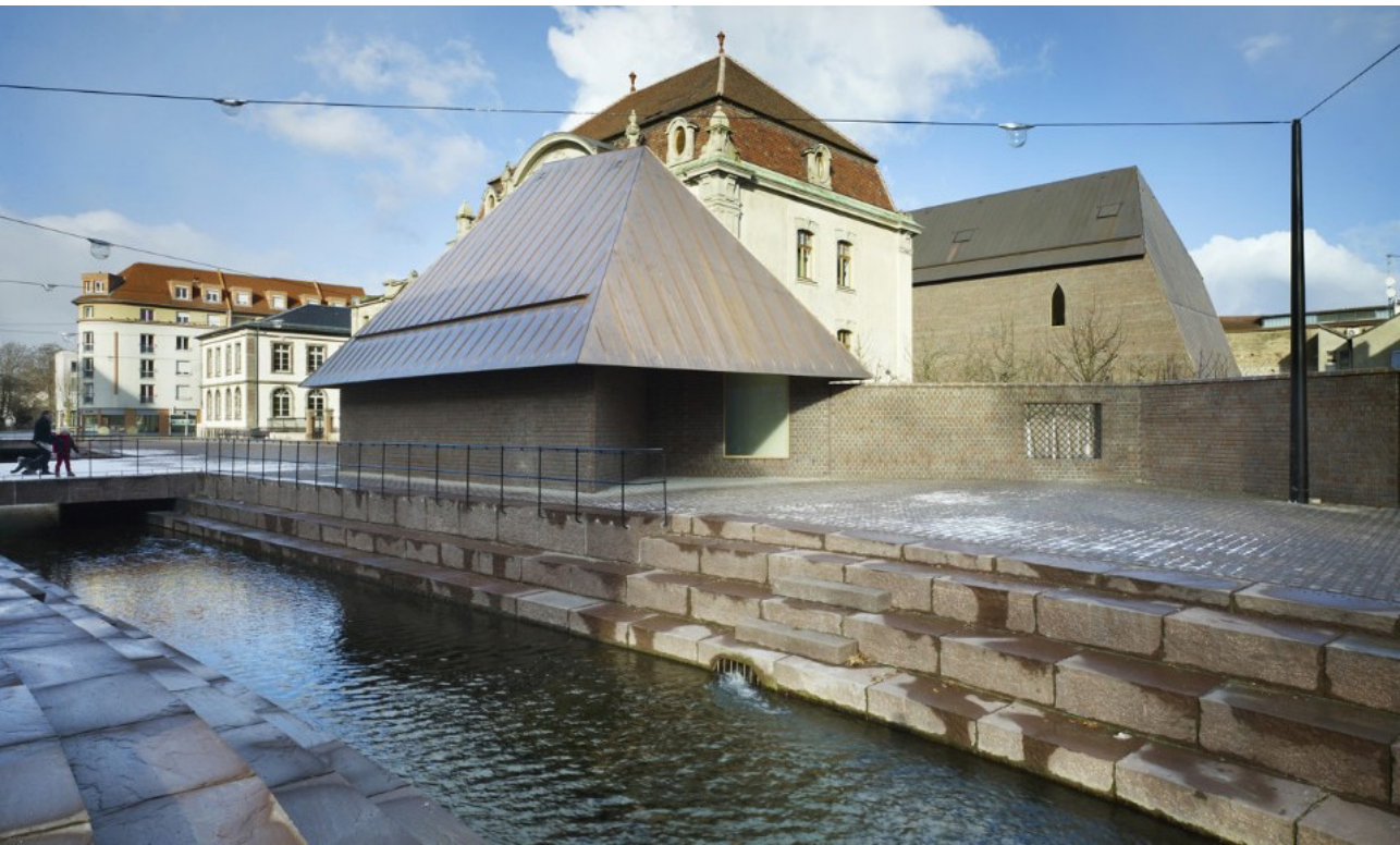
Figure 2.6: Musée Unterlinden Extension (2015), Herzog & de Meuron. As the positive environmental qualities are being recognized in recent years, several previously covered streams and rivers are being opened again for the public to enjoy.
