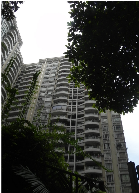
Figure 3.31: A typical residential apartment building in Guangzhou. For a limited budget, rounded balconies and varying roof shapes have become standard methods for the contour effect. Note also the lush vegetation in the courtyard of the building complex. Guangzhou, 29.07.2015
