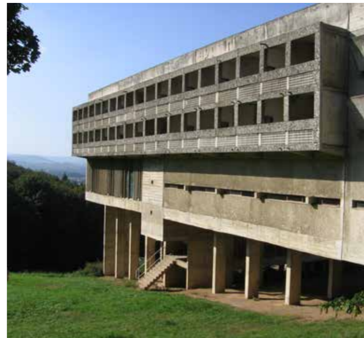
Sainte Marie de La Tourette, Lyon, France, built in 1960. A convent design by Le Corbusier as an example of Brutalism
