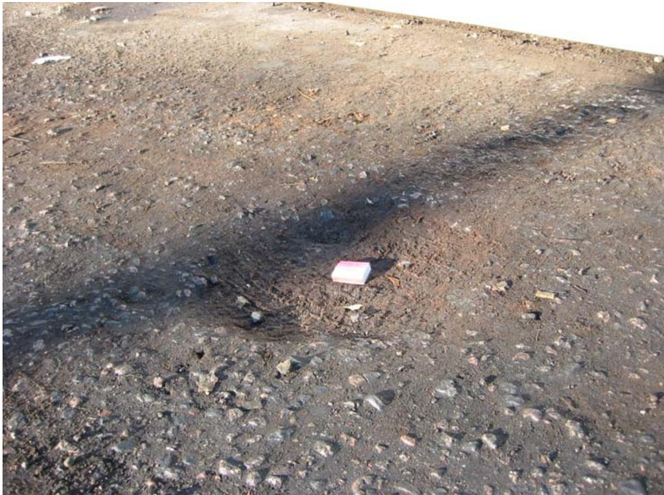
*Fig 5.1. A hole caused by fuel spillage on an asphalt forecourt pavement made of asphalt. Matchbox indicates scale.*
