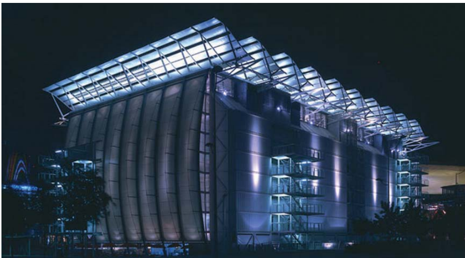
29 British Pavilion in Seville Expo. The facade with curved steel masts, spreaders and rigging with the stretched membrane skin. Nicholas Grimshaw Architects, 1992. (Jo Reid & John Peck/ www.grimshaw-architects.com )
