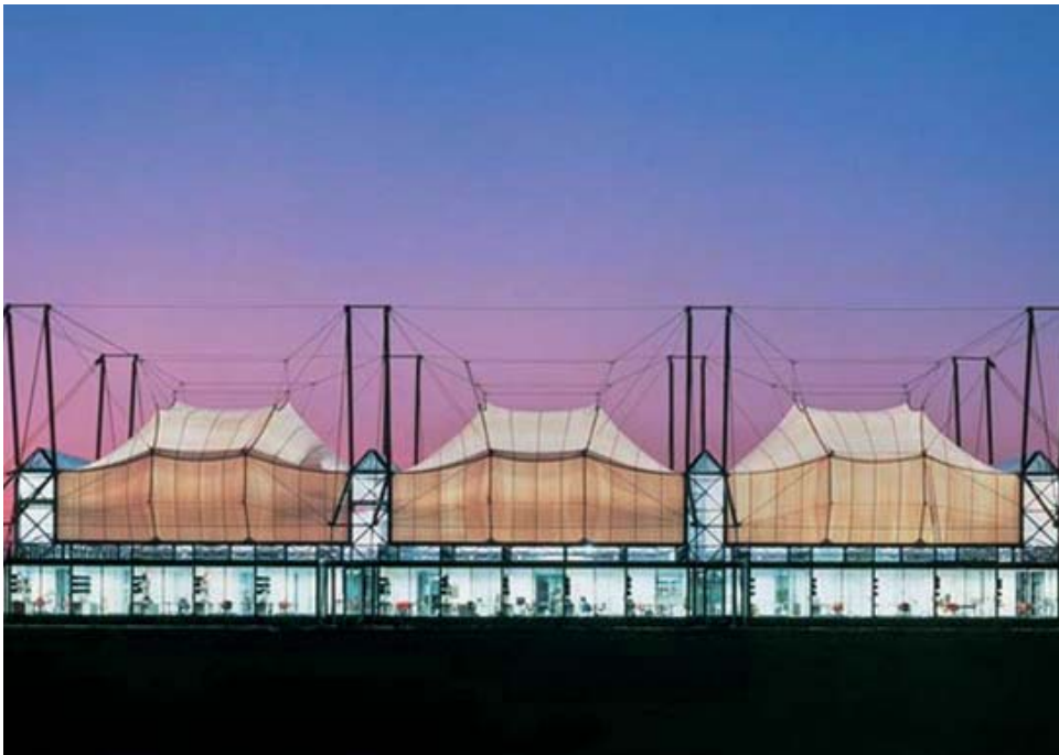
31 Schlumberger Research Institute at night. The membrane fabric roof reflects the light of the interior, thus creating a luminous element in the landscape. The office wings can be seen lit on the ground level of the building. ( www.hopkins.co.uk )
