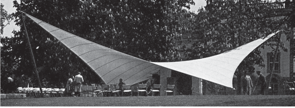
13 The four point double curved saddle shape structure of the Kassel music pavilion. Frei Otto and Peter Stromeyer, 1955. (Otto 1982, 64)
