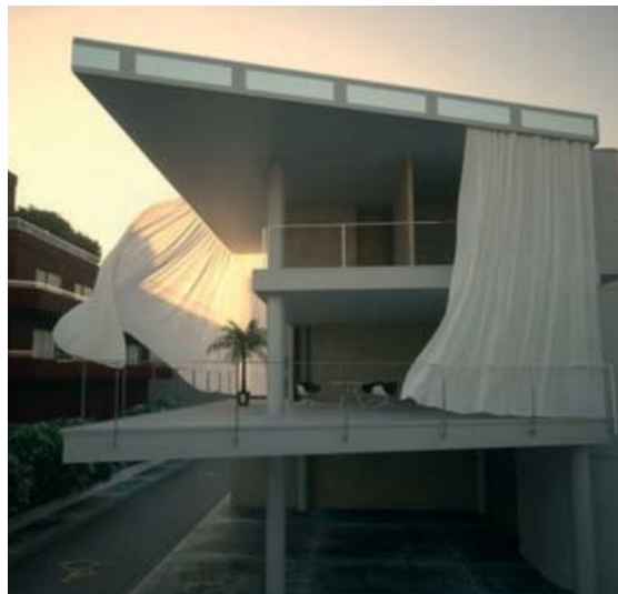
32 The Curtain Wall House in Tokyo. In the figure, the draping facade curtain clads the building like a dress. Shigeru Ban, 1995. (bakgård.blogspot.com 2008)
