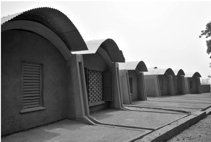
GANDO TEACHERS' HOUSING Diédébo Francis Kéré Gando, Burkina Faso, 2004
