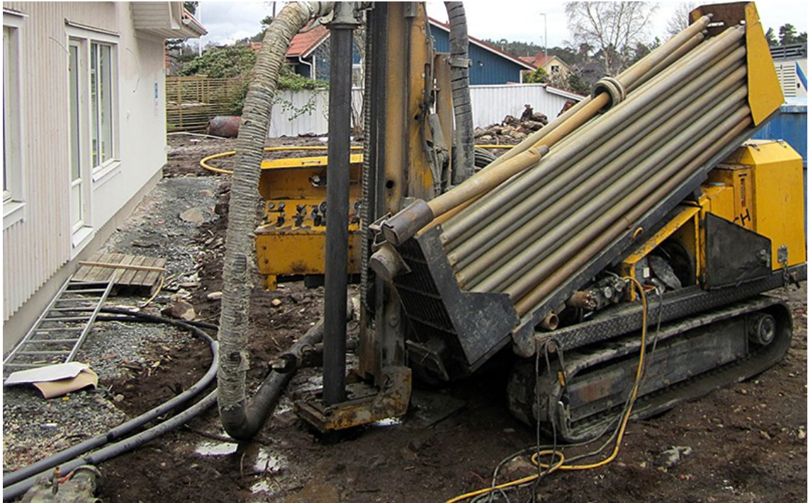
Figure 4. Well drilling rig [8]
