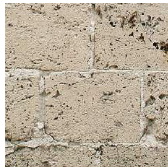
ITALIAN TUFF BRICKS Facades restauration.
