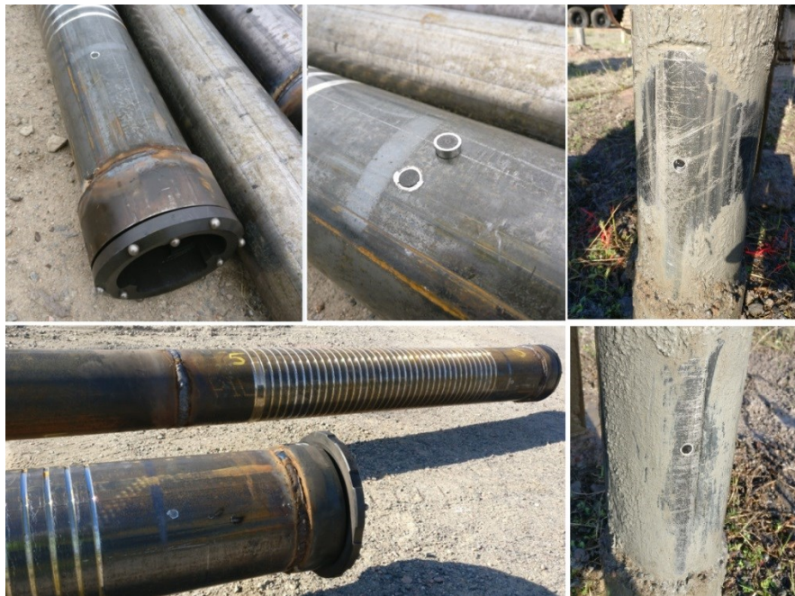
Figure 32. Grouting valves before and after drilling
