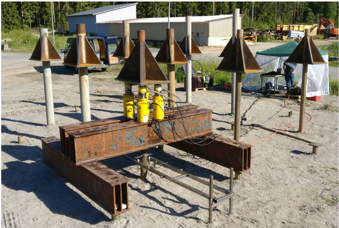
Figure 39. The loading structure and the test site
