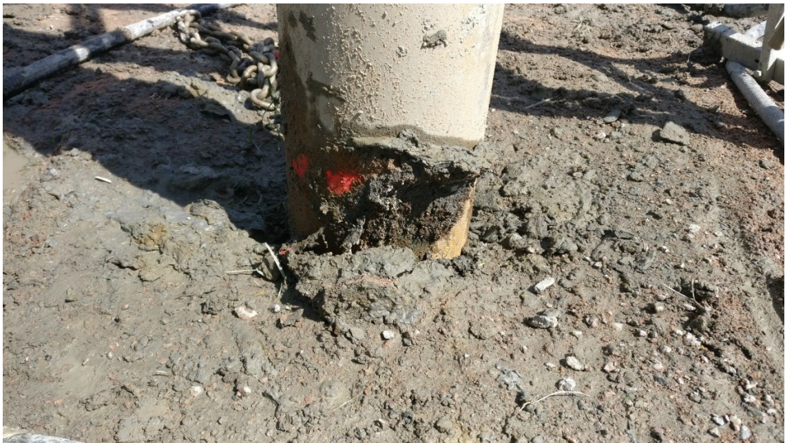
Figure 36. P6 RDs 220 pile which rose from the ground
