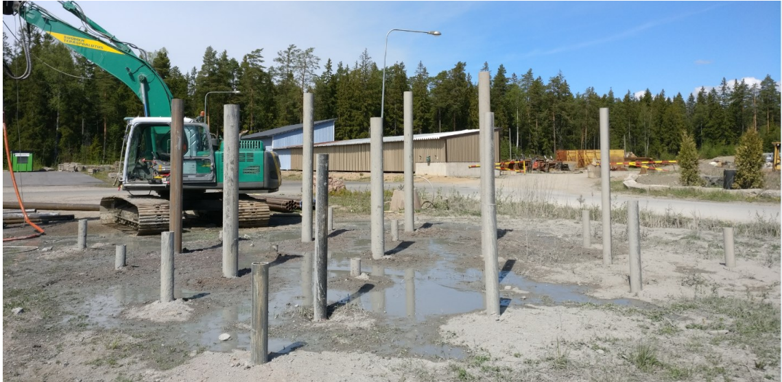
Figure 33. The test site after drilling
