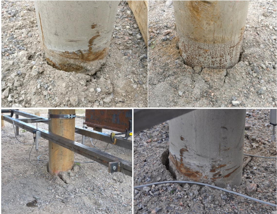
Figure 47. Displacements next to test piles after loading
