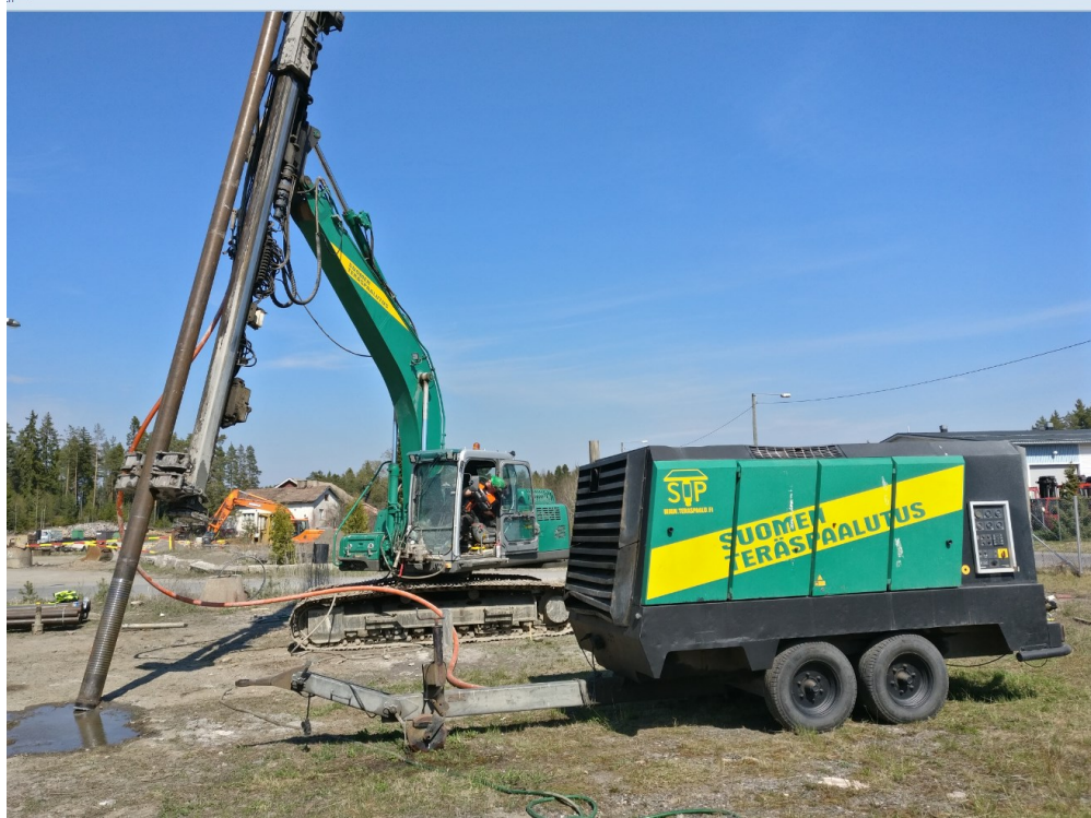
Figure 28. Drilling rig and compressor
