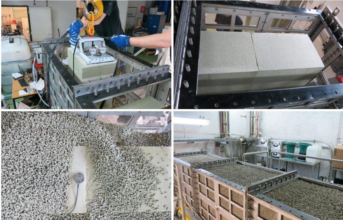
Figure 36. The floor of the tunnel was filled with a 95 mm thick pellet layer and six backfill blocks were installed into the tunnel with a vacuum lifting device. After the blocks were installed, the rest of the tunnel was filled with the pellets.
