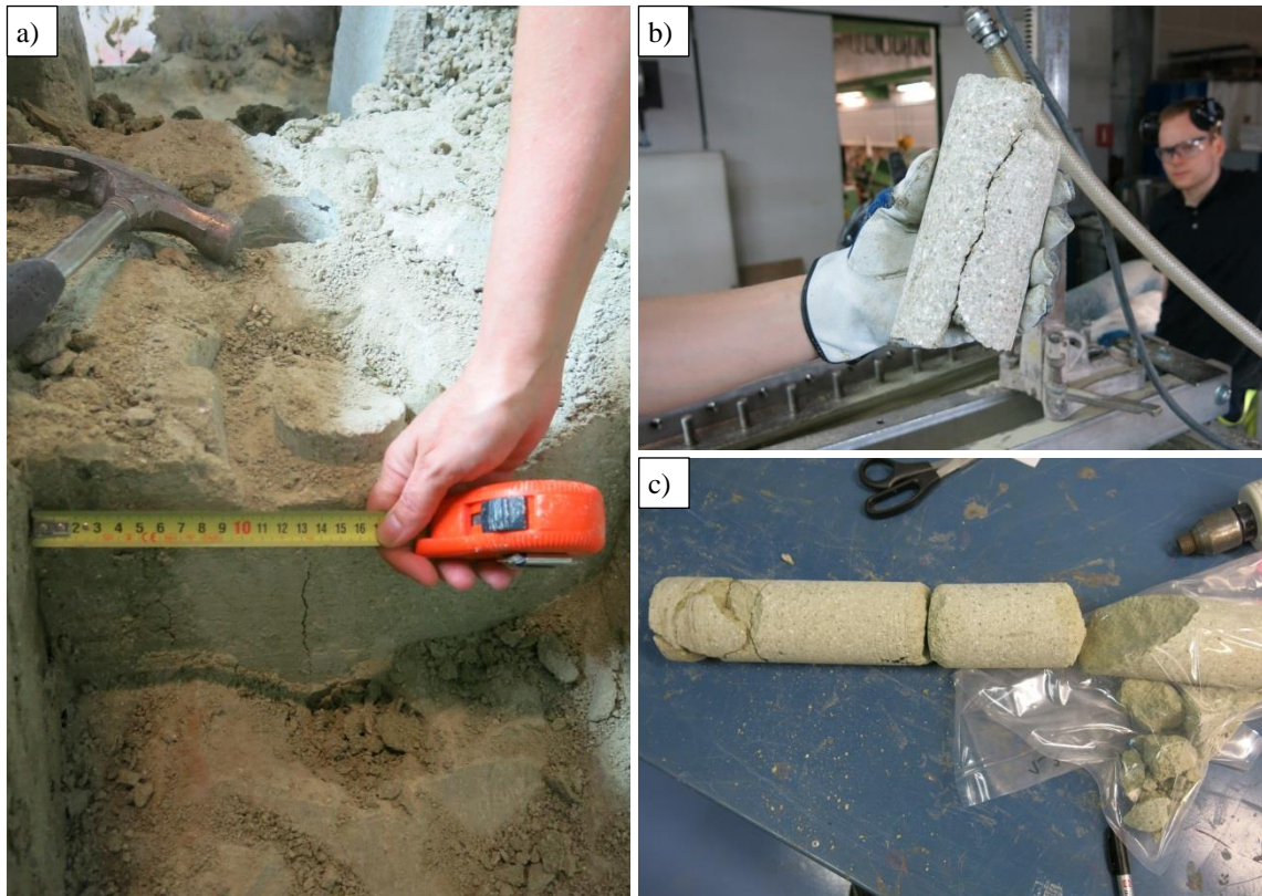
Figure 43. Backfill block cracks were found during the dismantling work: a) the backfill block 4 and its interface with the backfill block 3, b) drilled sample from the backfill block 6 next to the North end, c) drilled sample from the backfill block 3 which was above the buffer. The bottom side of the sample is on the left.
