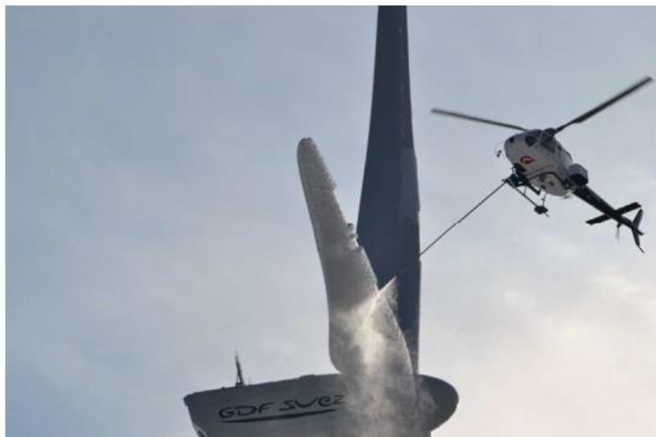
Figure 29. Ice removal with hot water sprayed from the helicopter. [86]
