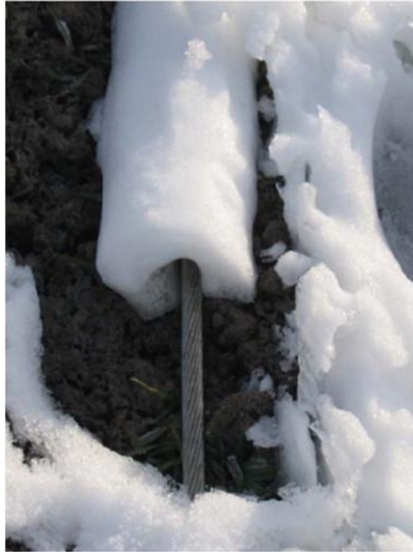
Figure 23. Wet snow accretion on the collapsed overhead line. [80]
