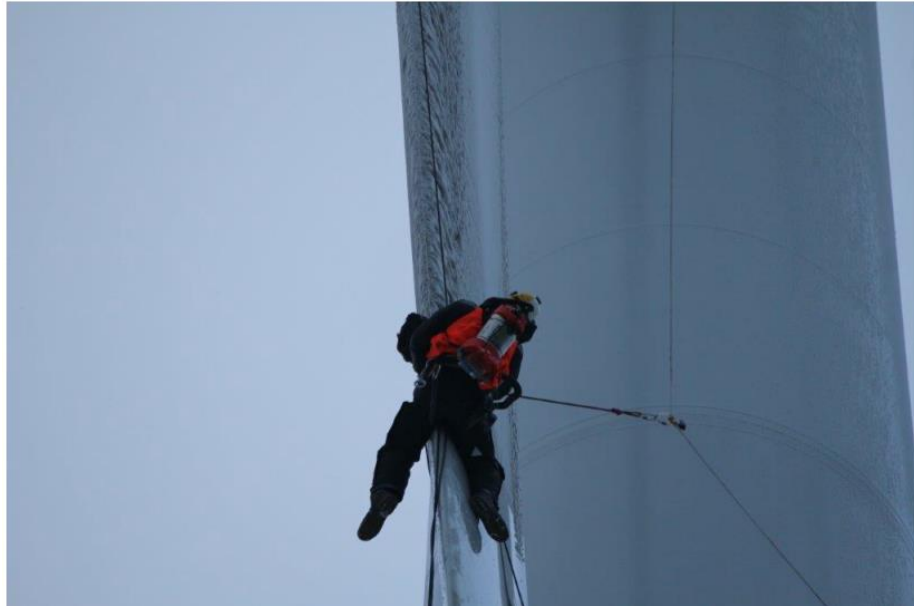
Figure 28. Manual ice removal from the wind turbine blade. [85]
