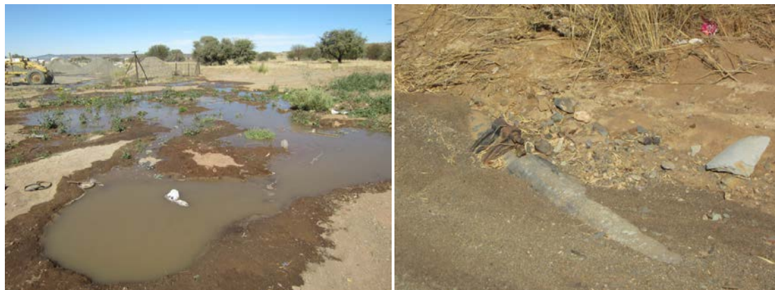
Figure 6.3. Leak in the industrial area was located in an hour since decrease of water pressure was reported (left) and a pipeline that is not protected (right) (Tuovinen)
