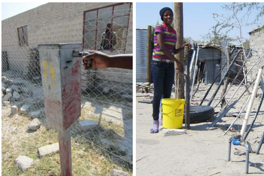
Figure 5.2. Non-functioning standpipe prepaid water meter (left) and a typical household conventional water connection in Ondangwa (right)(Tuovinen)
