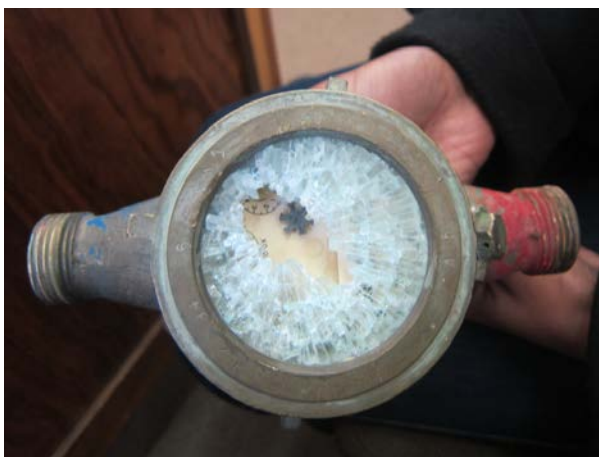
Figure 6.6. A resident of Keetmanshoop broke the water meter in hope to avoid water bills (Tuovinen)
