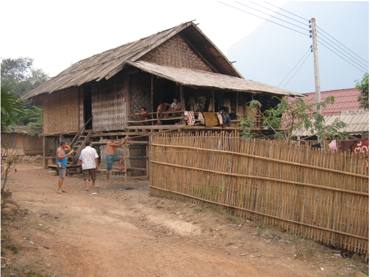
Photo 1: Wires connecting electricity to a house in Naseng
