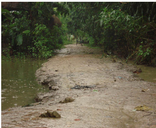
A clay road in Bangdom during the rainy season
