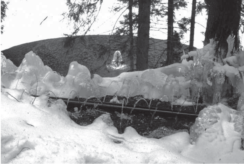
Figure 6. Water is pumped from the Lake Alajärvi to the Ahvenisto esker. Surface irrigation goes on despite of winter time. There is irrigation pipeline in front and one of recharging basins in the background. (Hämeenlinna Region Water Supply and Sewerage Ltd)
