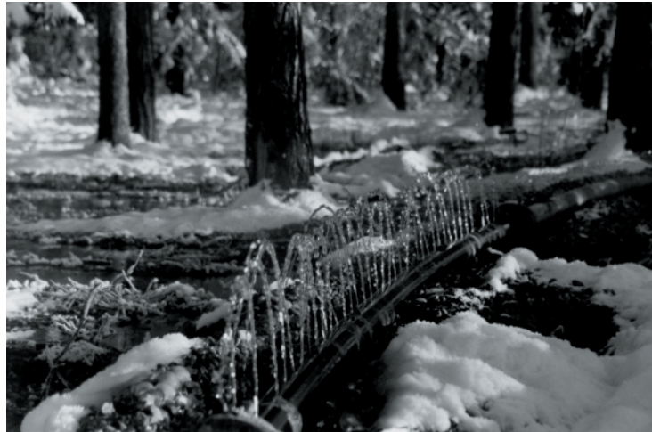
Figure 3. Use of spray irrigation as a recharge method in the Rusutjärvi area in 1998. (Photo: TSV)
