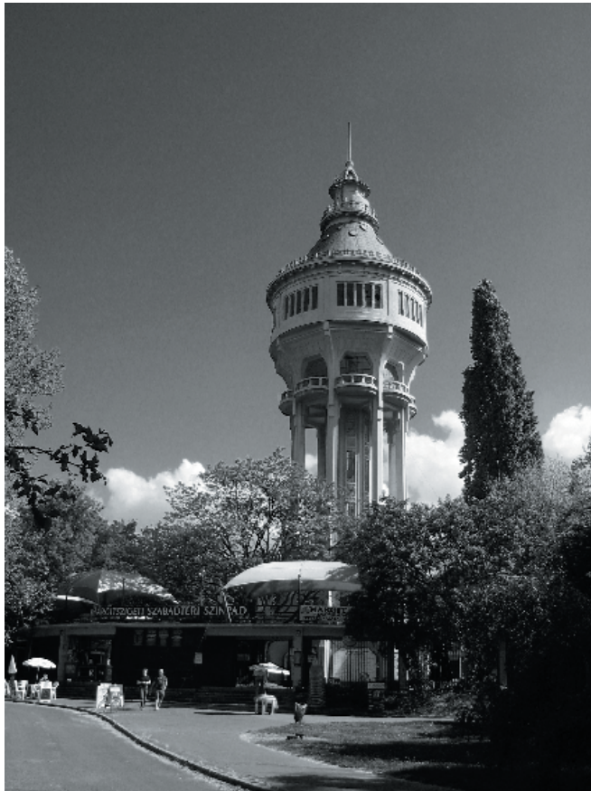
Figure. Water tower in Budapest, Hungary. (Photo: T. Katko 2005)
