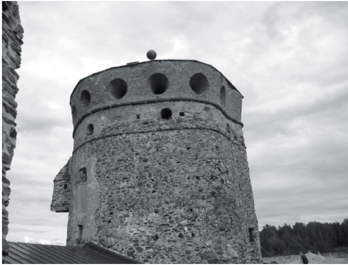
Figure 3. Bey privy attached to tower of Olavinlinna Castle, Finland. (Photo: P. juuti 2005)
