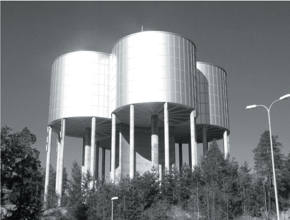
Figure. Water tower in Espoo, Finland. (Photo: T. Katko 2005)
