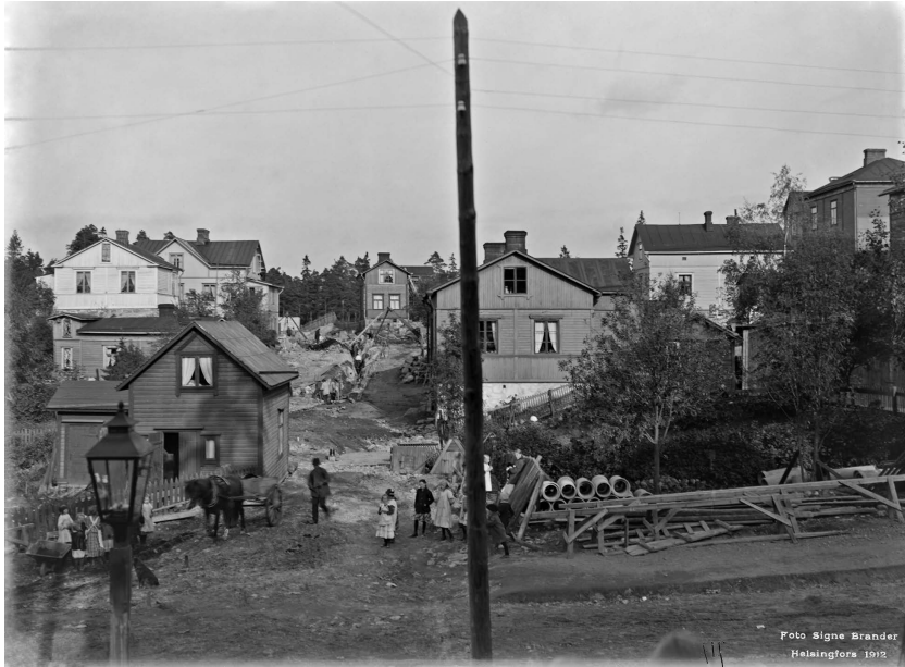
Figure 5.1 In 1912, following Fredriksberg’s annexation to the city, sewer systems were established in the area. A haphazard settlement layout with narrow streets posed a challenge to the installation of the infrastructure networks. Photo: Signe Brander, 1912, Helsinki City Museum.
