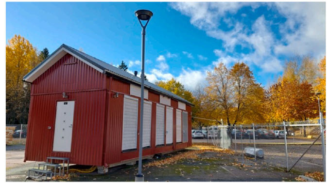
Fig. 2. View of test building 2 and surrounding terrain.
