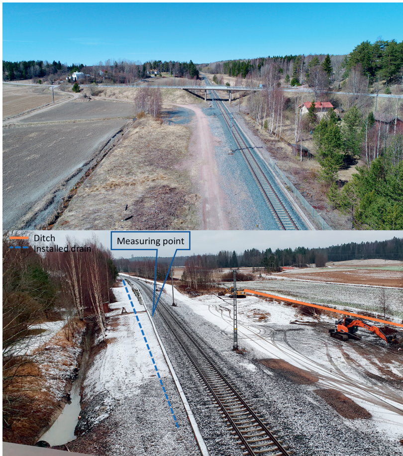
Fig. 2. The areal picture of Km 44 before and after the drainage improvement from opposite perspectives. The track is on flat terrain, and the drainage was not working properly. Photos taken on May 04, 2017, and January 29, 2020.
