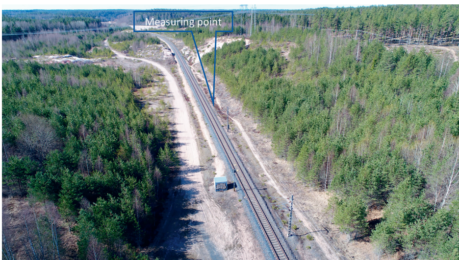
Fig. 4. The southwest areal picture of Km 137. The site is located near the sand esker that slopes in the direction of the track. Photo taken on May 04, 2017.
