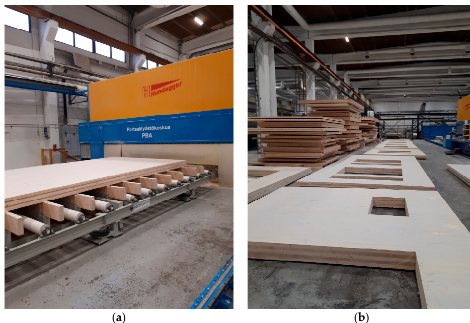
Figure 6. CLT plant: (a) view from the production line; (b) prefabricated building facade module produced (photo by authors).
