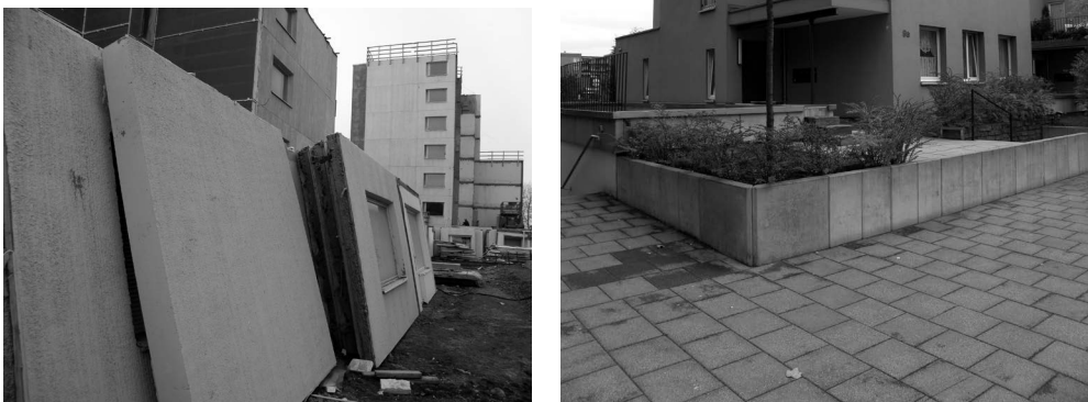
Figure 3.1 Concrete elements deconstructed from the buildings behind them (left). Location: Finland. A new building made from deconstructed elements (right). Location: Germany. Photos: SH.
