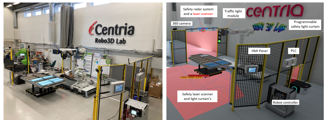
Figure 12. The demonstration production cell at Centria’s production automation laboratory and a digital twin of the cell. Presenting the configurable safety zones and the safety-approved devices monitoring the zones.
