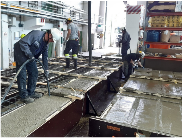
FIGURE 1 Casting of the test beams
